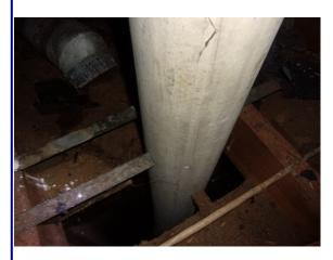
Another common area is **Transite** pipe which was used as exhaust ducts for HVAC furnaces. Transite is a cement compound that contains asbestos. In the photo to the left the pipe comes up from the furnace in the basement and exits through the attic. As with the tape, it can be painted over (encapsulated) and only becomes a problem when it becomes damaged and friable. Once friable you'll need an expert to remove it.
